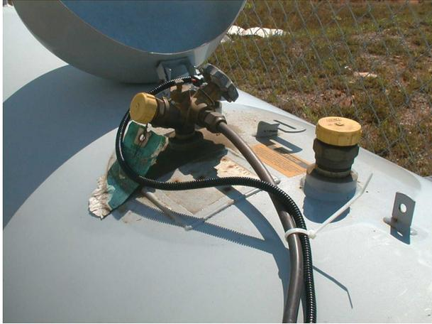
Figure 2. Monitor Installed on Tank
