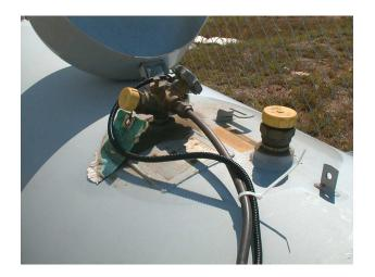
Figure 7. Monitor Installed on Tank
